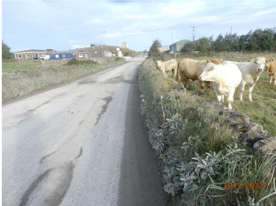
Figure 34: Access road through my lands is substandard in width for quarry traffic
