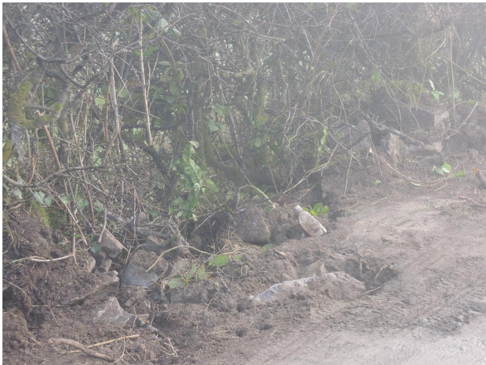
Figure 39: Destruction of boundary drystone walls and hedging, removal of roadside grass margin (January 2024)
