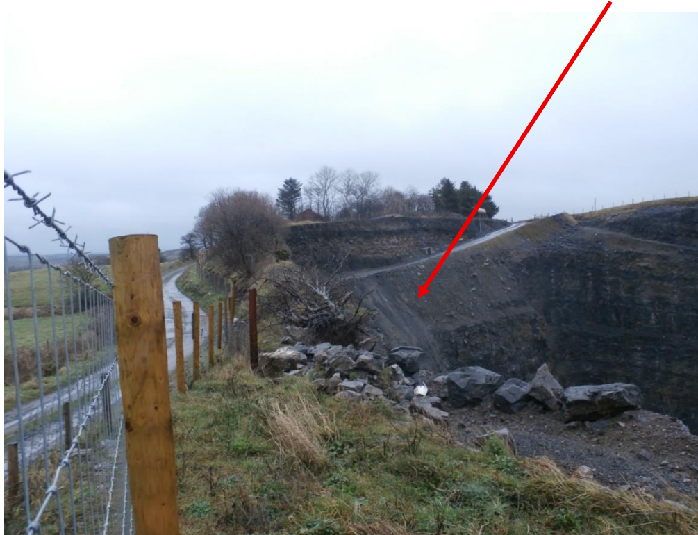
Figure 11: Photograph from 07 th January 2015 showing evidence of waste material dumped over face of north quarry
