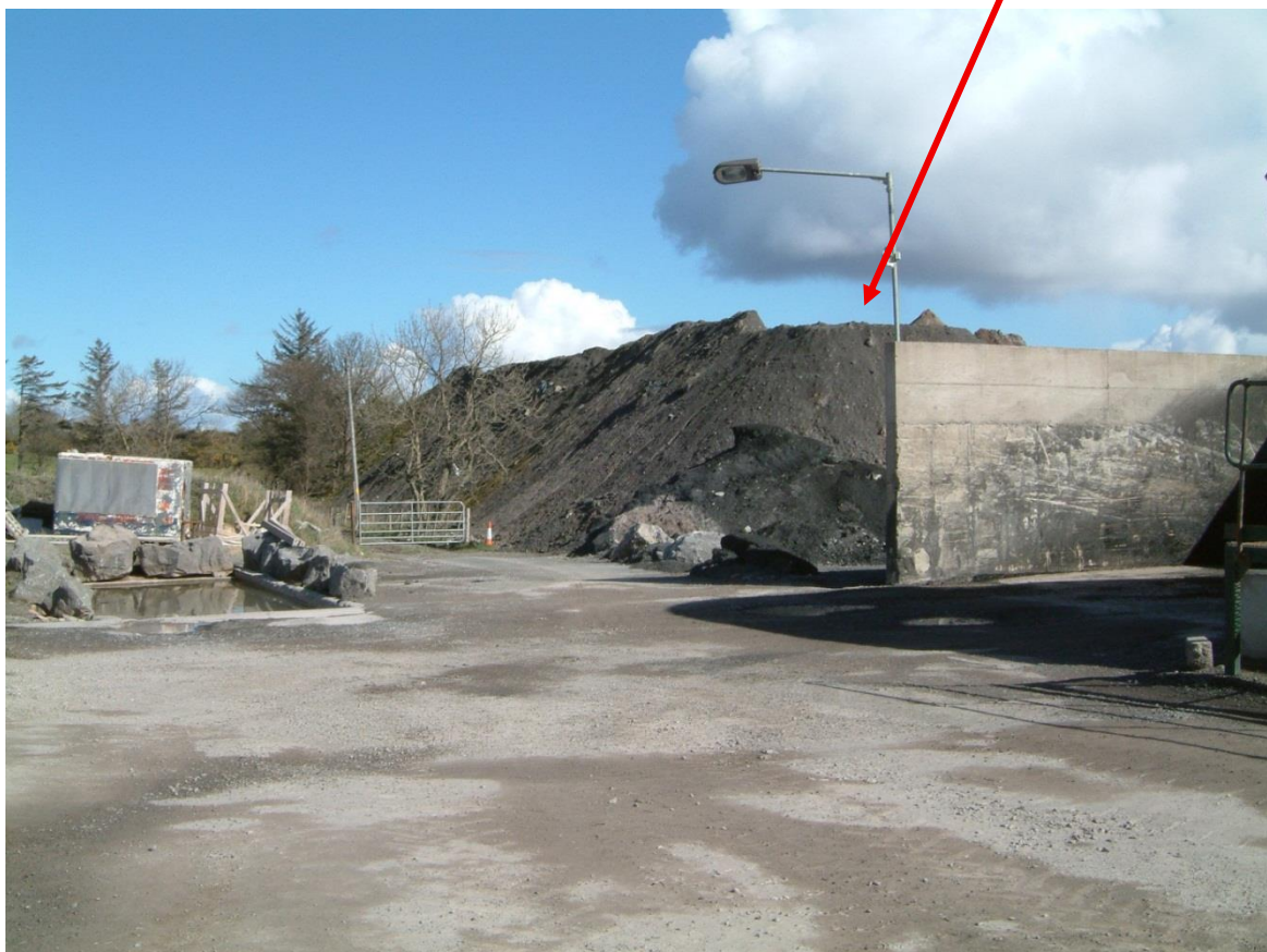
Figure 8: View of stockpile of waste material taken from publicly accessible road - March 2012
