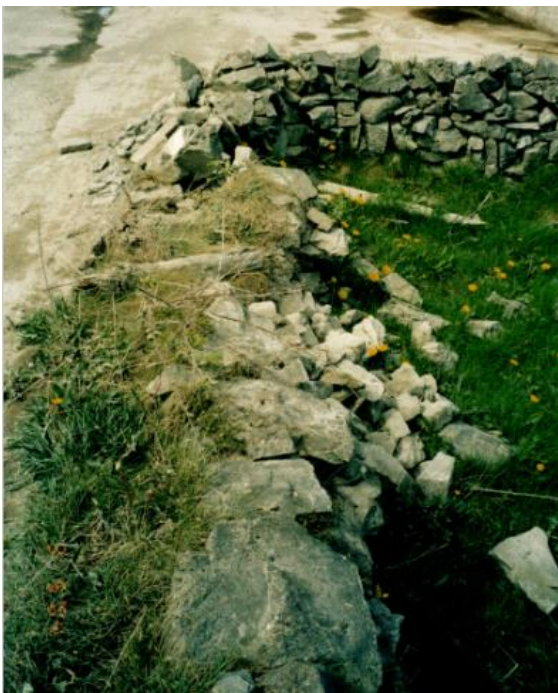
Figure 33: Damage to drystone walls with stones falling into field creating hazard of cattle escaping
