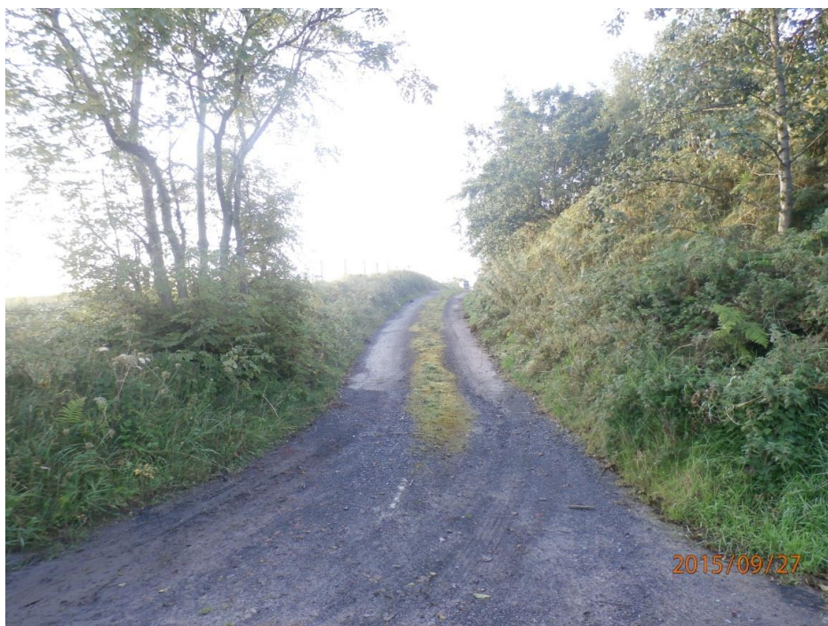
Figure 35: Northern section of access road through quarry at junction with L7265. This section of road is not subject to quarry traffic and shows the character and width of the original road
