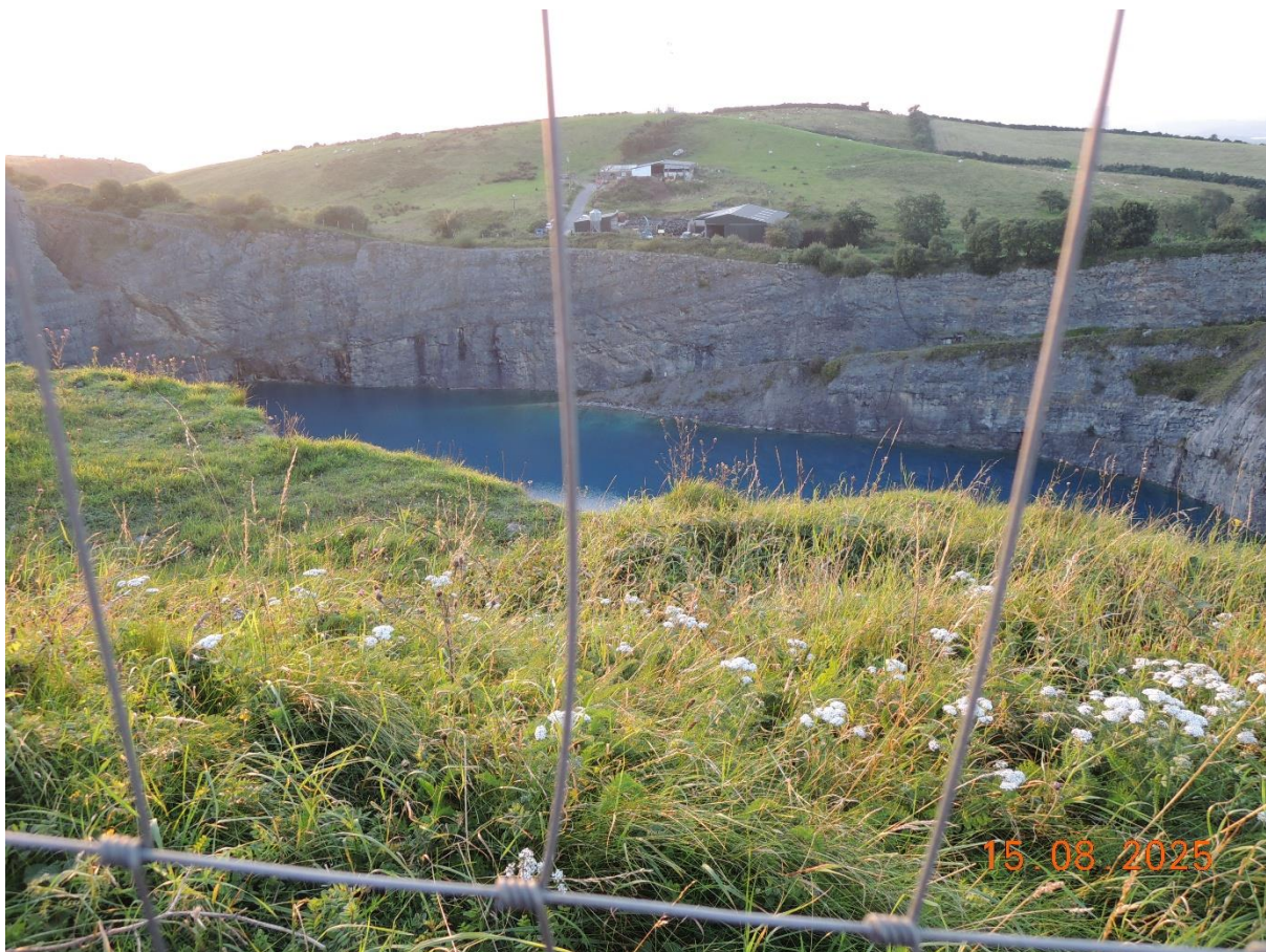
Figure 27: Inner face of berm sloping towards cliff edge
